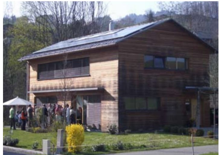
A PassivHaus in Austria – this house incorporates some passive solar features such as south facing glazing and also external shading devices, but the overall build format and internal layout is not necessarily that different from a standard house.
