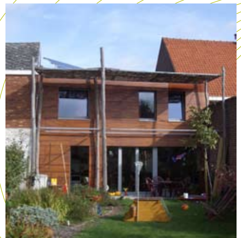
PassivHaus - Private residence in Oost-Vlaanderen Belgium
