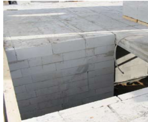
Aircrete block and plank
