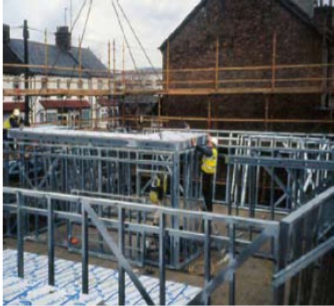
Panellised steel frame
