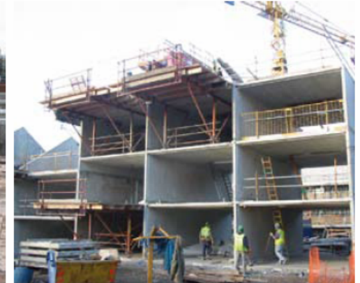
Tunnel form construction
